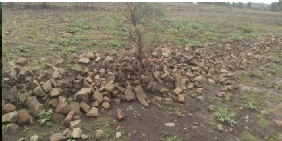
Terrace demolished due to rodent
