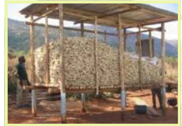
Figure 16: Good storage structure raised on poles with metal plates wrapped around the poles against rats
