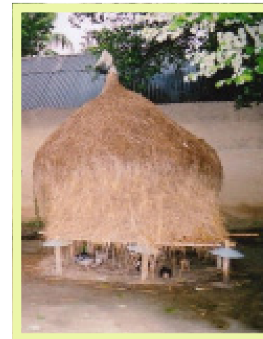
Figure 17: Example of rotational disk at the poles to prevent rats to climb up
