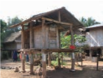
Typical grain store within a rural village, Laos. Note the metal sleeves to try and prevent access by rats. The grain is stored loosely in the woven bamboo structure. Photo: Alex McWilliam (CSIRO)
